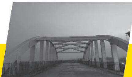
OPEN WEB BRIDGE GIRDERS
